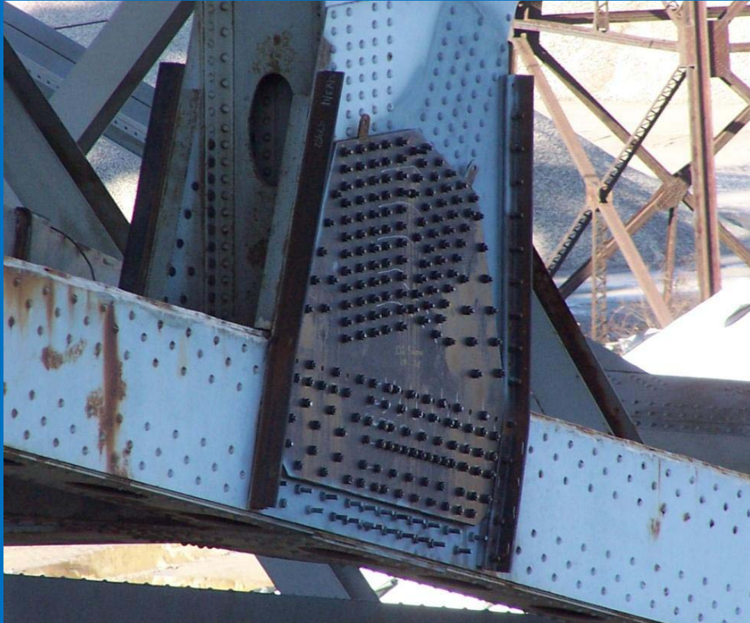
Adding Plate and Edge Stiffeners
